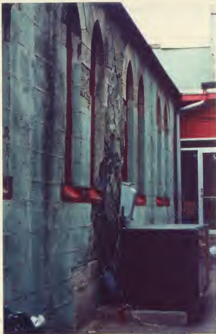
South Elevation of Church Building (U)
